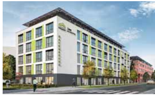
Ravensburg Abb.: I-Live (in Bau)
