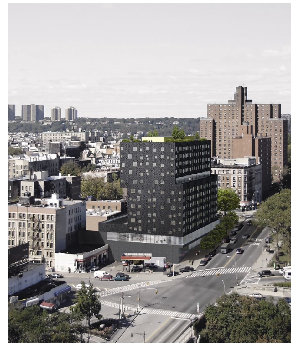
Sugar Hill, 404–414 West 155th Street, Manhattan | geplante Fertigstellung 2014
