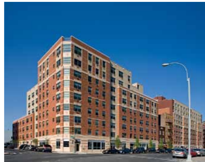
Parkview Commons I (2007), 406 East 161st Street, Bronx
