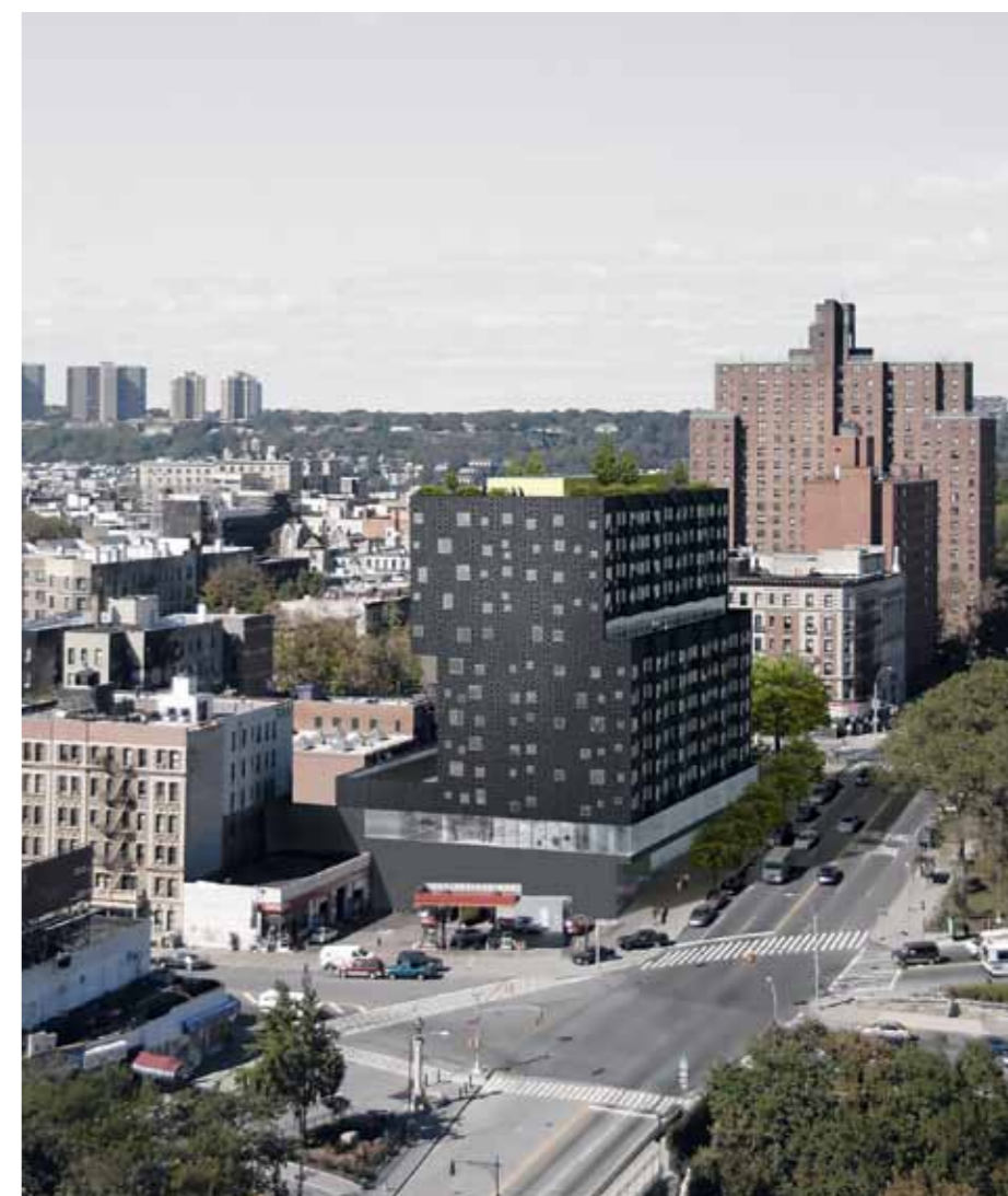
Sugar Hill, 404-414 West 155th Street, Manhattan | expected date of completion 2014
