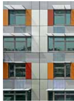
View from the east: The façade was assembled from pre-fabricated panels complete with sunshades and balconies. The materials include wood, cement, and aluminum.
