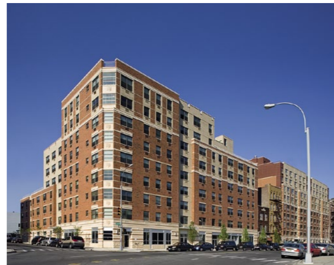
Parkview Commons I (2007), 406 East 161st Street, Bronx
