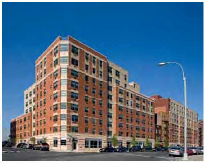
Parkview Commons I (2007), 406 East 161st Street, Bronx
