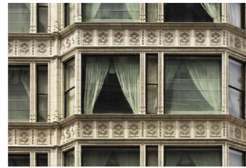
Reliance Building | Foto: Florian Fischer
